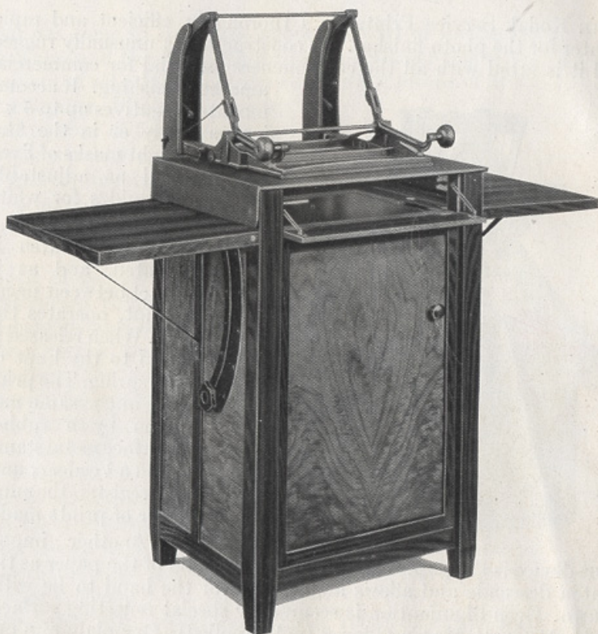
Eastman Professional Printer showing Vignetting Door open
